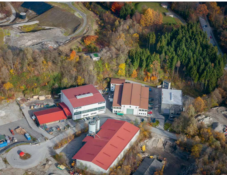
Facility in Turkey
